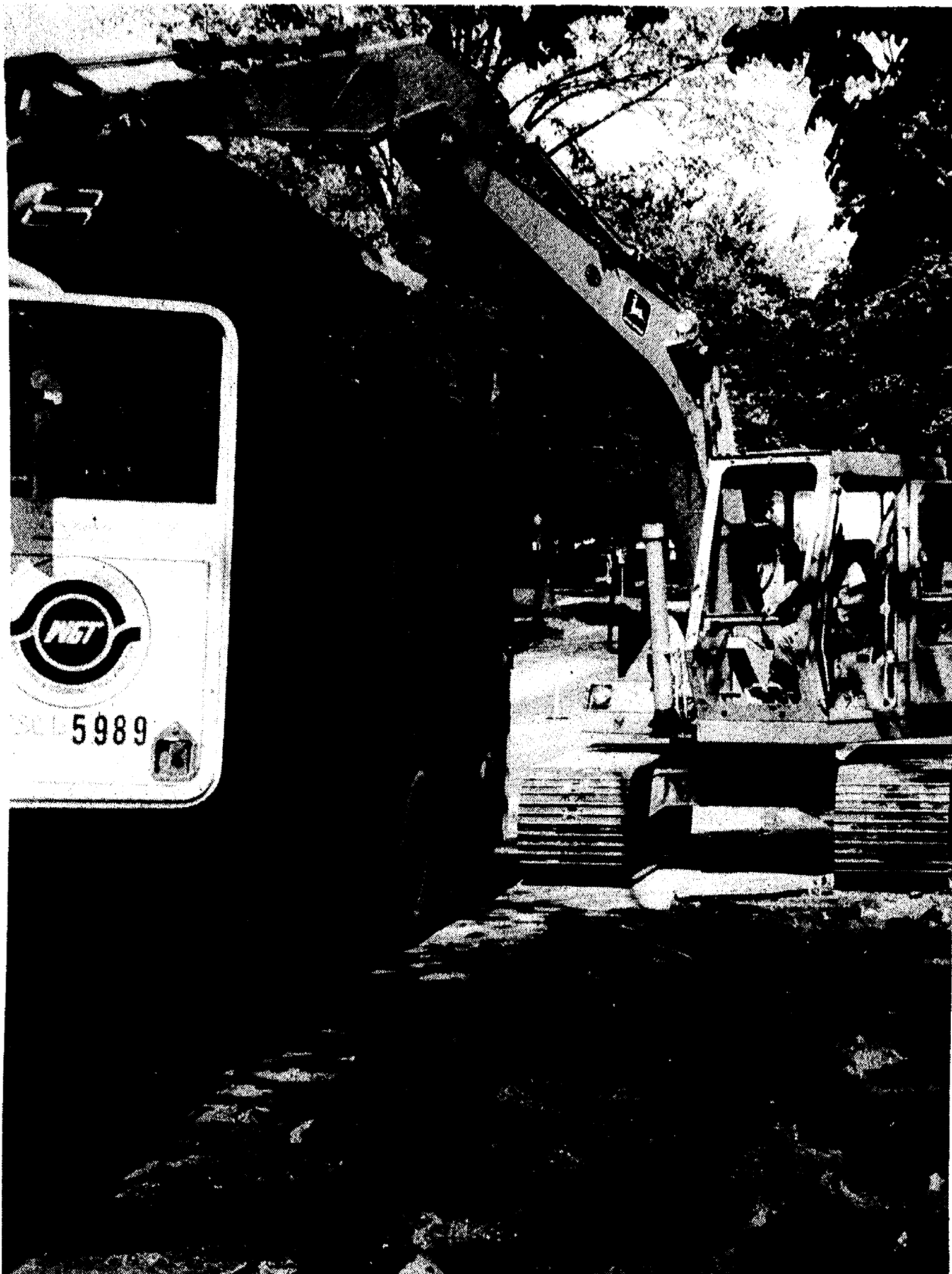
OLD CURB is being dug up along M-52 and being replaced by new curb at a fast clip as part of a project that will involve M-52 from the hospital on the south to Sibley Rd. on the north. The state is completing the work and the
